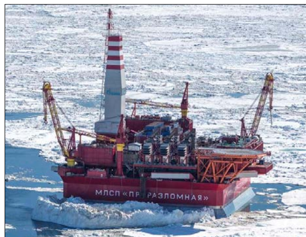
Figure 20. Sea ice pile-up around Prirazlomnoye caisson structure (source: Gazprom Neft Shelf LLC)
