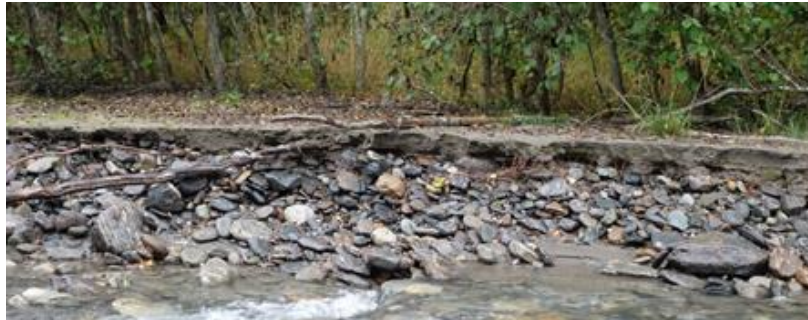
Figure 79: Photograph of a 70 cm high river bank located on the Russedalselva river. The bottom section of the river bank is dominated by cobbles and the top 15 cm consists of well sorted medium sand. Photograph taken on 19 September 2016 (location shown in Figure 77).
