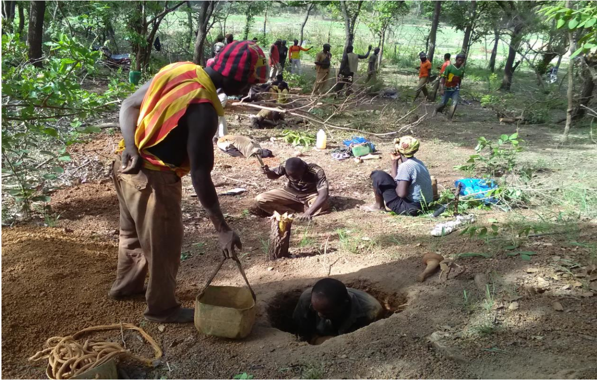
Figure 3: Yacouba's team starts with pit digging
