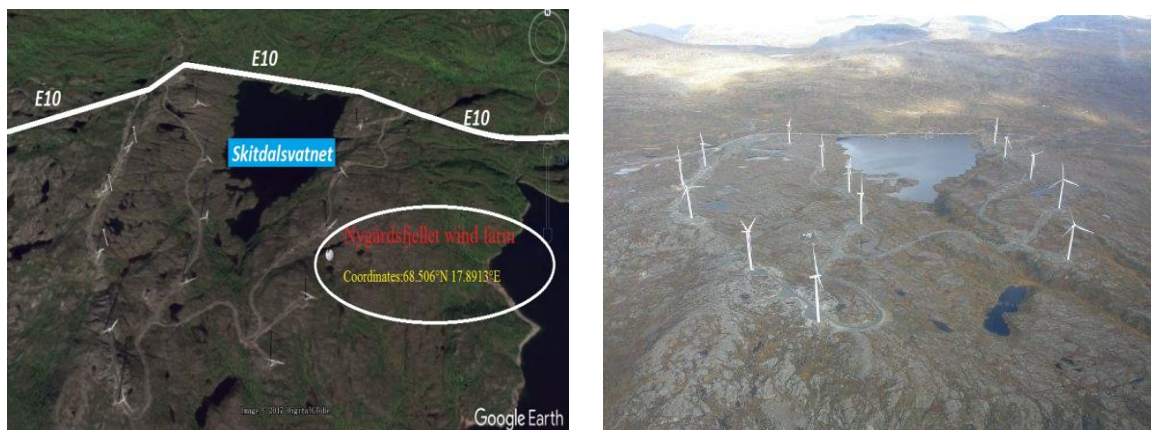
Figure 1-2 Terrain overview of Nygårdsfjellet wind park
