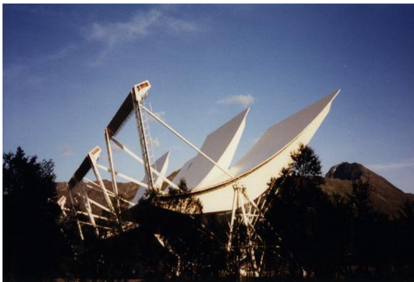
Figure 3.1 → Tromsø 224MHz radar.
