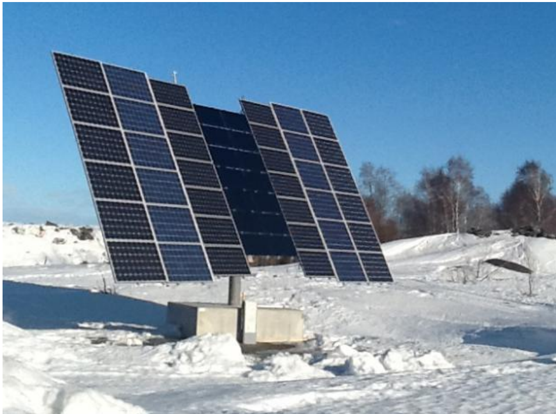
Figure 2-7: Picture of a two-axis tracking system in Piteå, Sweden. (Christensen 2012)
