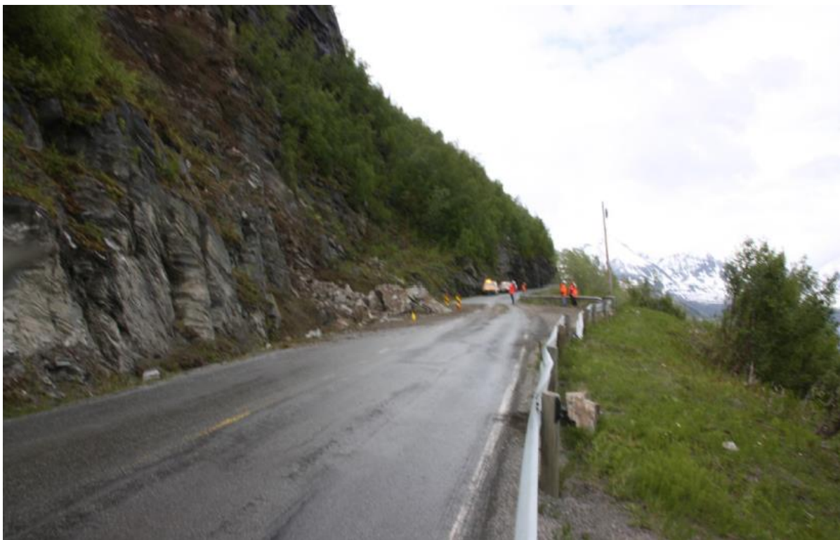
Figure 35: Boulders on the road after the 2014 rockfall. From (Vegvesenet, 2014b).
