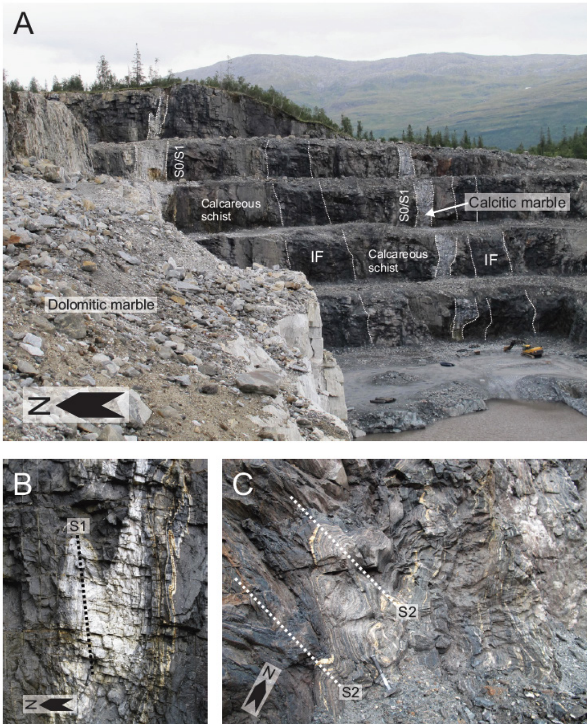
Figure 16 – Photographs from the Kvannvatnet open pit mining area illustrating the main structural features of the ore-bearing Dunderland Formation. (A) Eastern wall of the open pit exposing the steeply dipping main ( S_0/S_1 ) foliation of the various rock types, including dolomitic and calcitic marble, calcareous schists and iron formations (IF). (B) An isoclinally sheared dolomitic marble unit typified by steeply south-dipping axial planar ( S_1 ) surfaces (scale of photo is c. 4 m in height). (C) East-facing wall exposing asymmetric, open F_2 -folds with N-dipping axial planar surfaces ( S_2 ) in an Mn-enriched zone.
