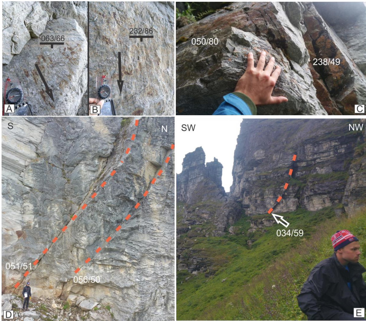
Figure 19 - A + B: Slickenlines (station 6). C: Conjugate set with orange coating (station 1). D and E: Joints with listric geometry (station 8).
