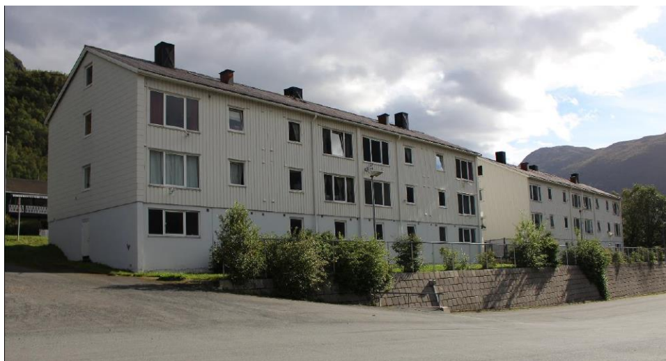
Figure 16. The case study building - Beisfjordveien 88
