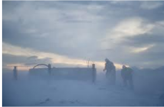
Figure 6. Unclear visibility in Fakken wind farm due to snowy weather conditions (ingun, 2013)
