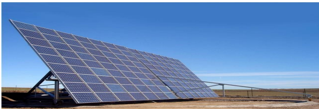
Figur 2.4.2 Azimuth-Altitude Dual-Axis Solar Trackers [11]
