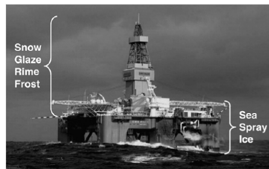
Fig. 2. Potential ice accretion areas on a rig (Ryerson, 2011).
