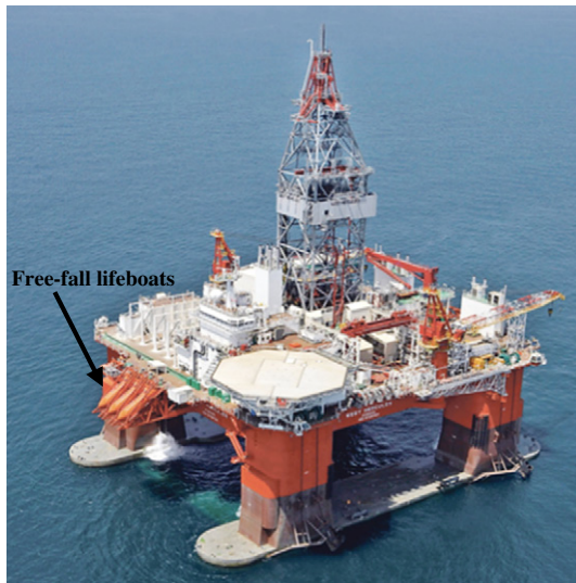
Fig. 6. West Hercules drilling rig used by Statoil in the Johan Castberg area, equipped with free-fall lifeboats (Seadrill, 2015).
