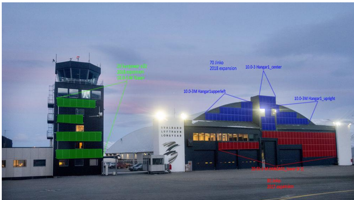
Figure 18: Location of five of the arrays that track production data
