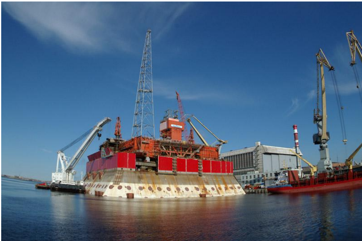
Figure 28. 'Prirazlomnaya' oil rig construction site. Source: www.sevmash.ru
