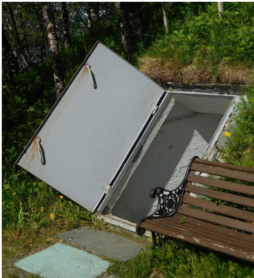
Figure 14: Entrance to the bunker housing the exhibition about the Tirpitz at the Tromsø Forsvarsmuseum. Photograph taken by Juliane Bockwoldt, 2016.
