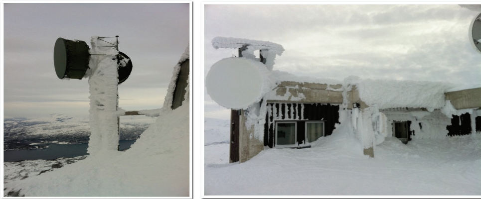
Figure 2: Ice accretion on communication devices and towers on Fargnesfjellet near Narvik, Norway
