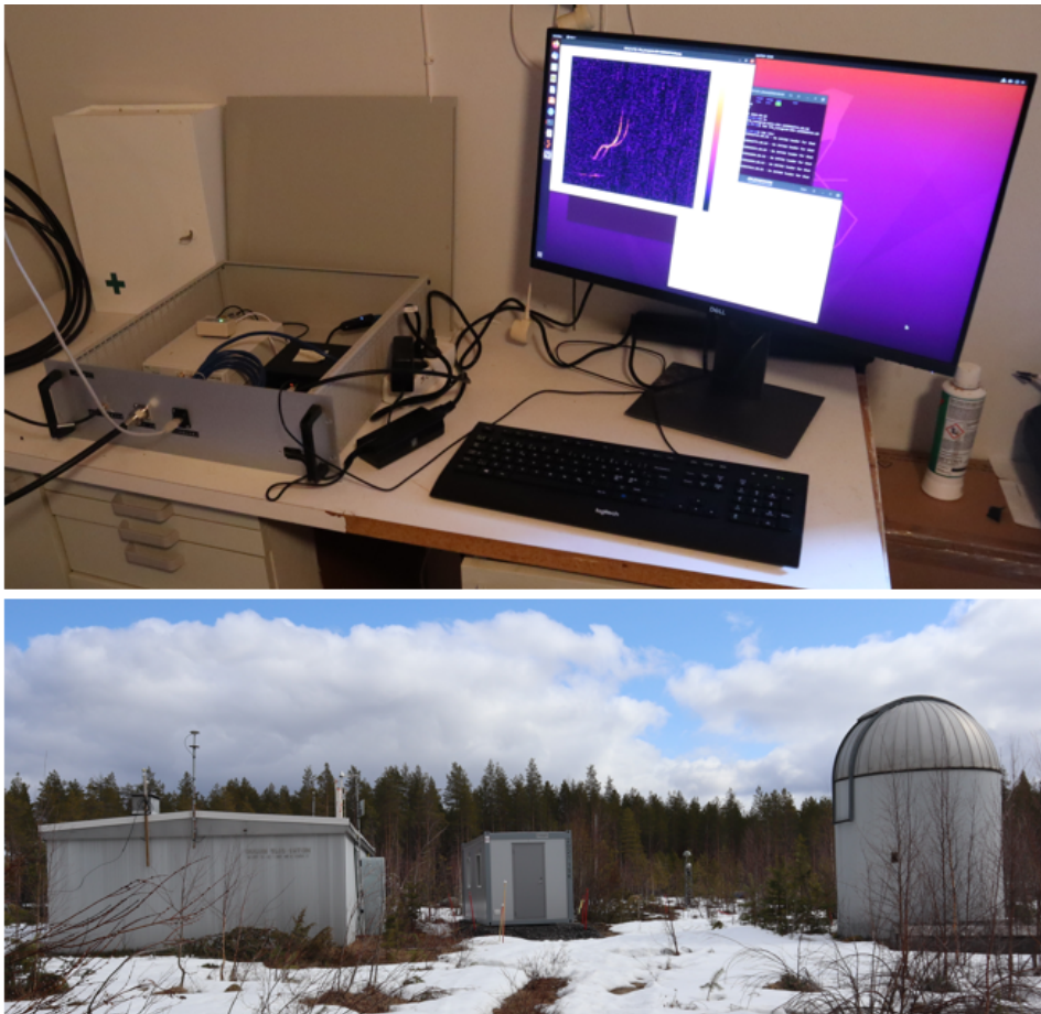
Figure 6.5: Rack mounted case for the Oulu site, photo taken during the setup of the instrument (top). Instrument shack on the Oulu observatory site the radar receiver was installed (bottom).
