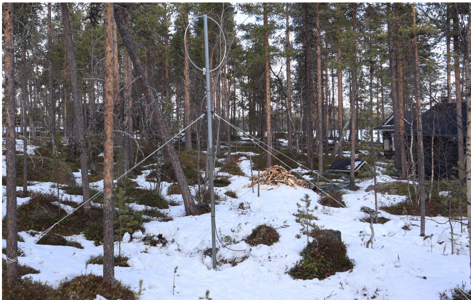
Figure 6.8: Photos of the antenna as it was installed on the Ivalo site. Trees were used to attach all four guy-wires.
