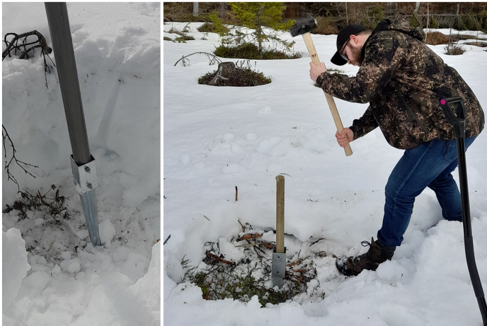
Figure 4.3: An image demonstrating how the bottom tube segment will be bolted to the earthen anchor after it has been driven into the ground (left). Using a sledgehammer, the anchor is driven far enough into the ground so that only the square part of it is revealed (right).
