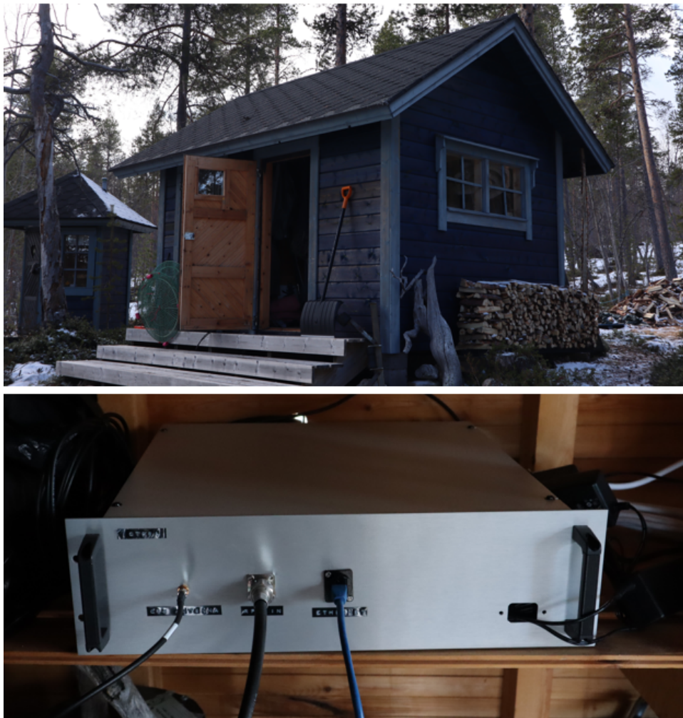
Figure 6.9: Photos from the Ivalo site. Rack mounted case inside the fishing shed (bottom) and the fishing shed located on the cabin property (top).
