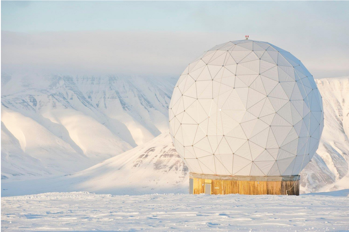
Figure 3. Svalsat antenna with radome covering (Anon., 2022)
