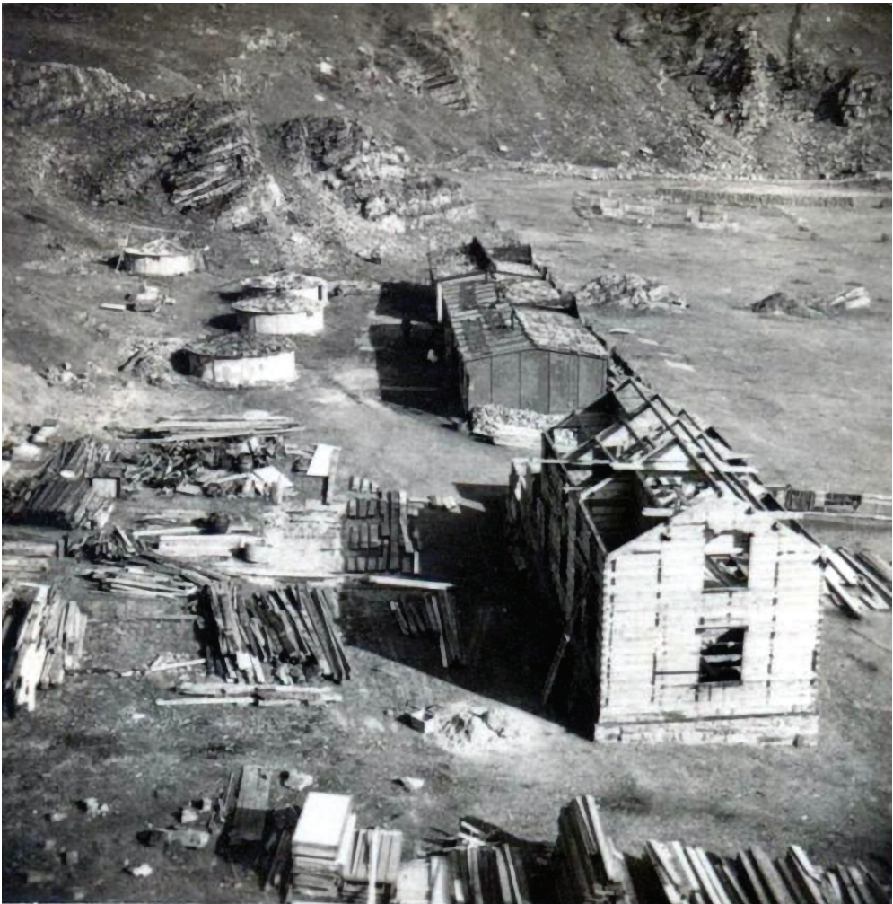
Figure 14. A) 1942 image of the German garrison under construction in the Sværholt village. Note the plywood tents in the back that were later used as midden-pits after the POWs were moved to the camp in Eidsbukta. b) Photo of the same area today. Photo: Unknown German soldier, and Bjørnar Olsen.
