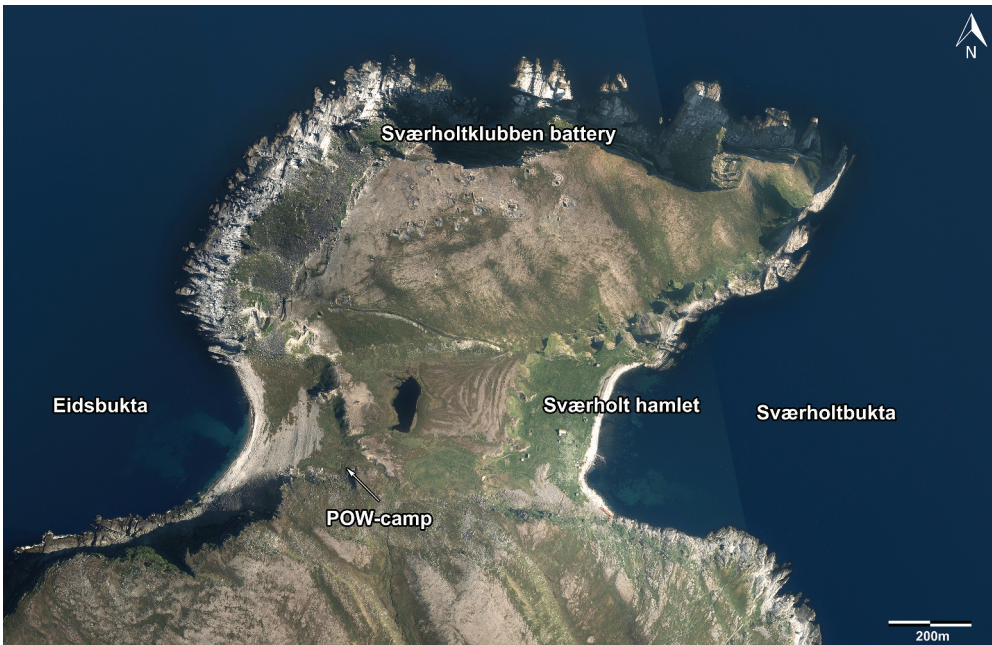
Figure 2. Aerial photograph of Sværholt from June 2018. The battery foundations, bunkers and remains of the blockhouses are discernable at the northern summit of the cape (Sværholtklubben). Photo: The Norwegian Mapping Authority. Illustration: Stein Farstadvoll.
