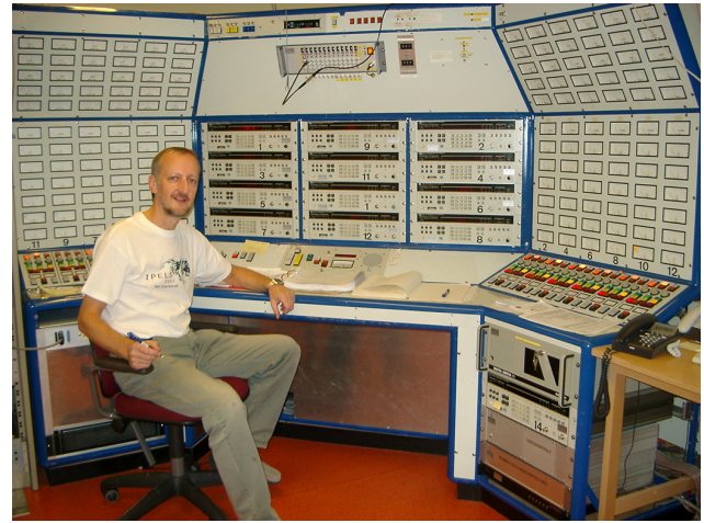
Figure 6. The Heating facility console in the control room as it was in 2007, with the first author at the controls. Six columns of meters, lights, and push buttons on each side show the status and are used to control each of the 12 transmitters. The 12 commercial RF synthesizers in the middle of the console have been replaced by digital synthesizers in the transmitter hall, and the space is now filled with large computer screens. (Photo credit: Michael T. Rietveld)
