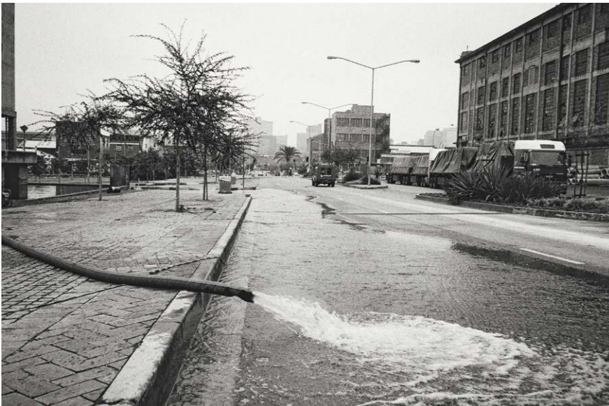
Figure 10 Water reservoir being emptied onto a street in Johannesburg
