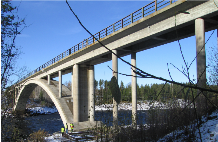
Figure 1: The concrete arch railway bridge over Kalix river in Långforsen.
