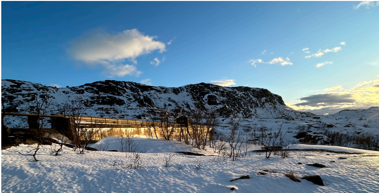
Figur 13. Jernvassdammen under befaring. (Foto: I.E.A.Hjallar, Feb. 2023)
