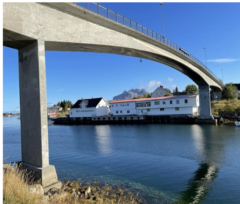
Figure 2. Picture of Herøysund Bridge built in 1966.
