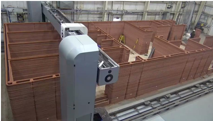
Figure 1: Construction of CHAPEA [10]
