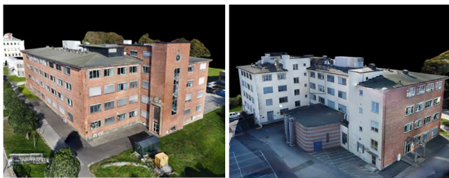
Fig. 2. 3D model of the building generated using photogrammetry
