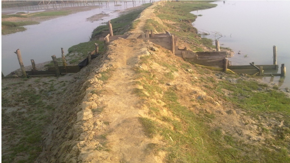
Figure 14: Dam and sluice gate of extensive shrimp farming
