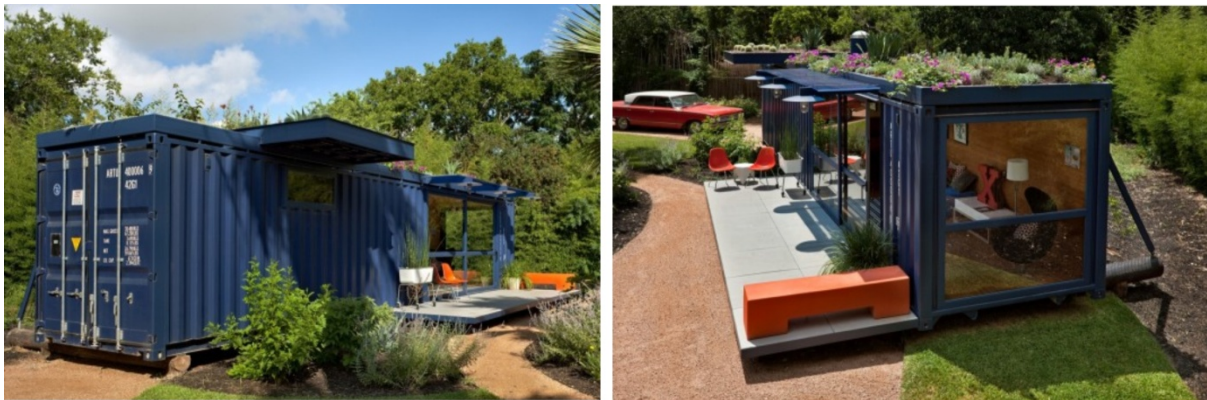
Fig.12 Shipping container is converted to the guest house by Poteet Architects, USA, 2010
