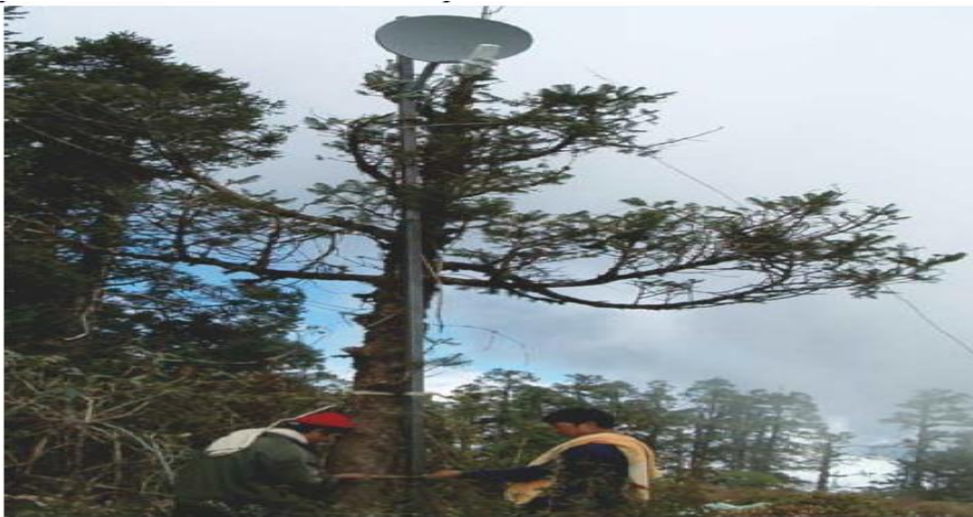
Figure 17:Using tree to place antenna grid 86
