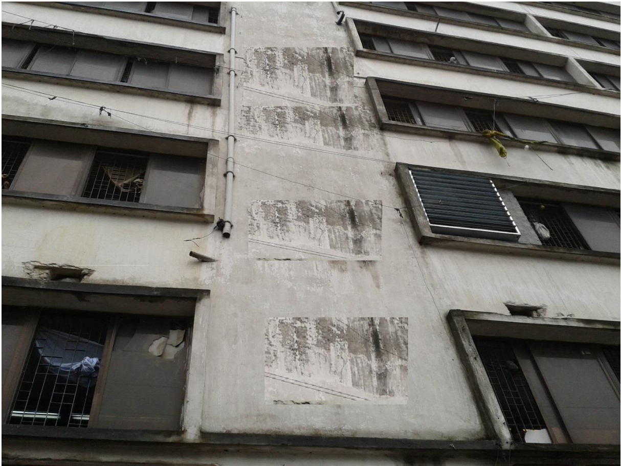
Figure 3: Garment factories in different floors of the building. The research informants work in these garment factories. I wanted to take pictures of the working environment but I was not allowed to go inside.
