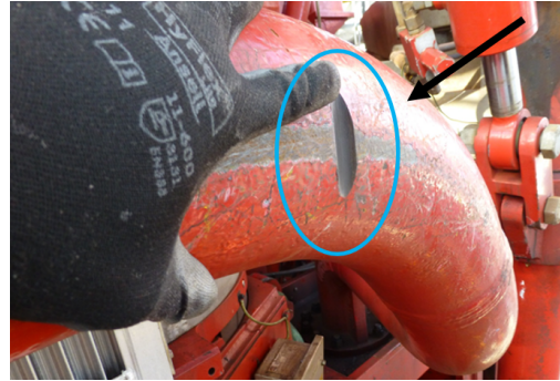
Figure 5.6: S-pipe with external wear.
