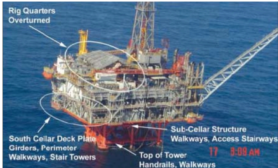
Figure 26: Complex cellar deck on the structure Pentronius that would accumulate ice easily if located in colder waters (Ryerson(b), 2008, p.24).
