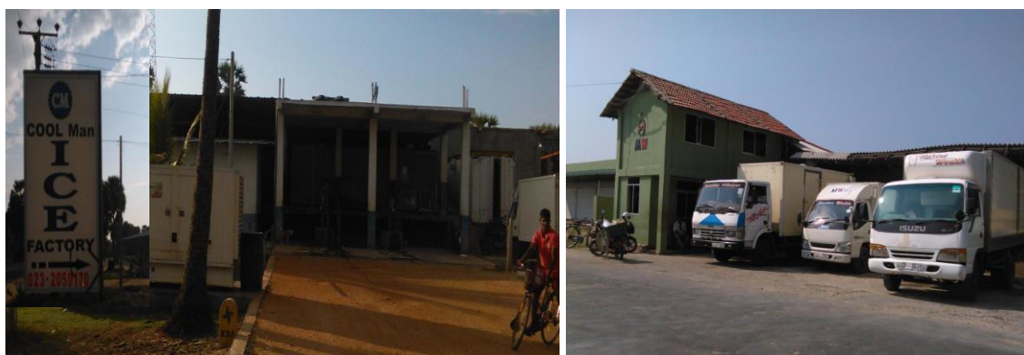
Figure 21: Available Ice plant facilities in Mannar (left) and Jaffna (right).
