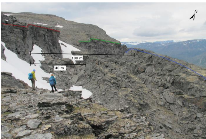
Fig. 22 Photograph showing the width, 100m, between the back fracture scarp (red lines) and the front block (blue lines), an accumulated displacement of c. 40 m in association to the cross-fracture scarp (green lines).
