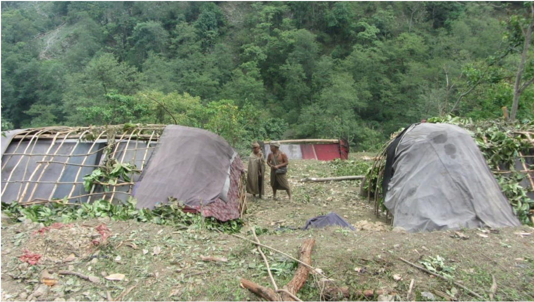
FIGURE 7, ONGOING CONSTRUCTION OF HUTS
