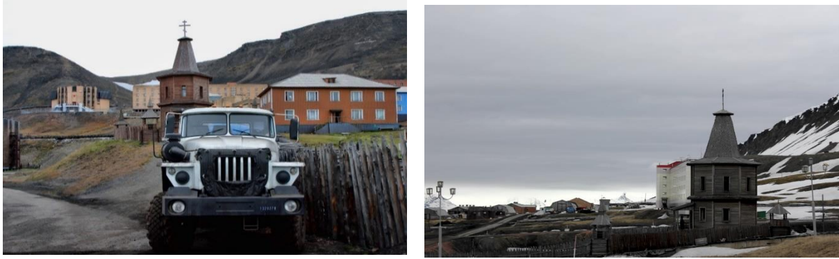
Figure 6. Barentsburg before the modernization 8 9
