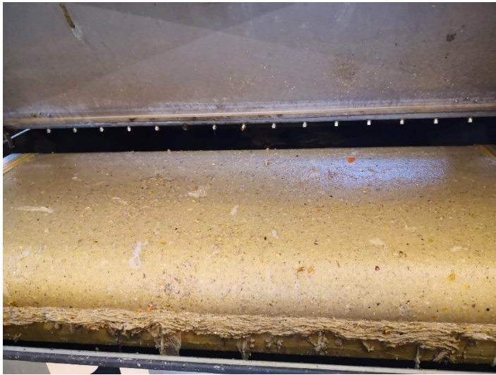
Figure 8. Filter mat at Breivik WWTP (private photo)
