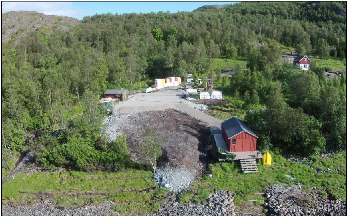
Figure 55: Photo of the groundwork associated with cabin building in 2015 (Photo: Vidar Heitmann).
