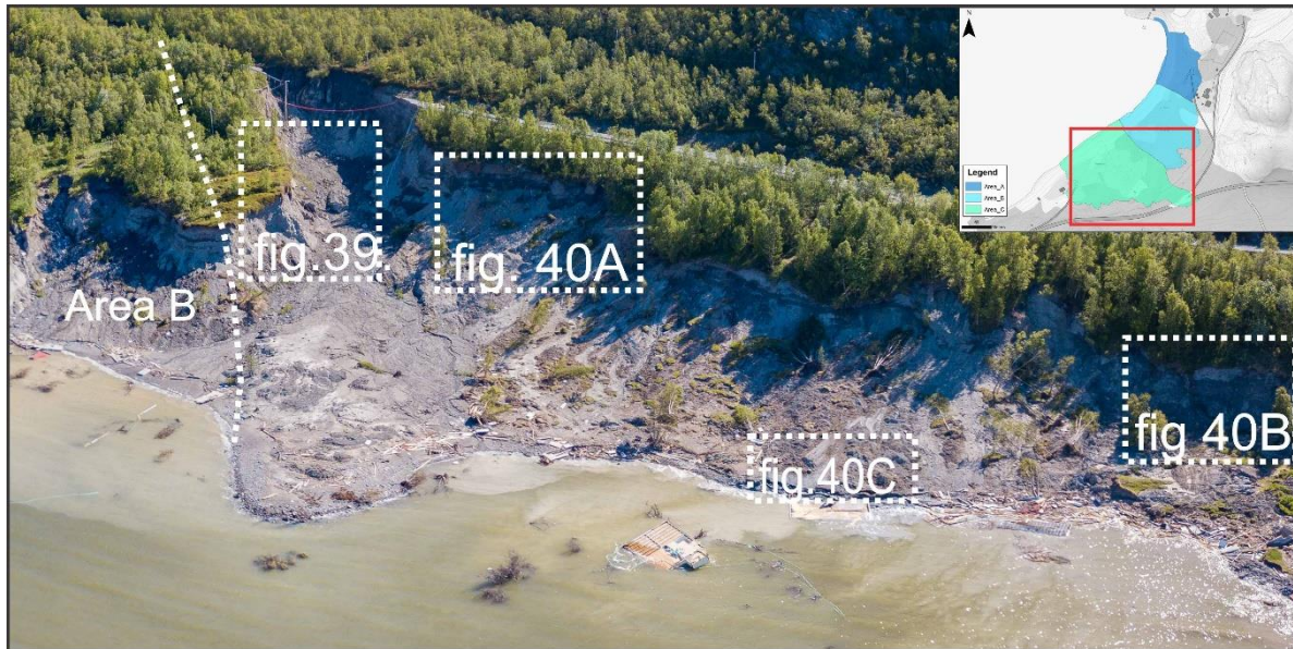
Figure 38: Overview photo from area C. White boxes illustrate the location of figures 39 and 40. Photo: Raymond Eilertsen .
