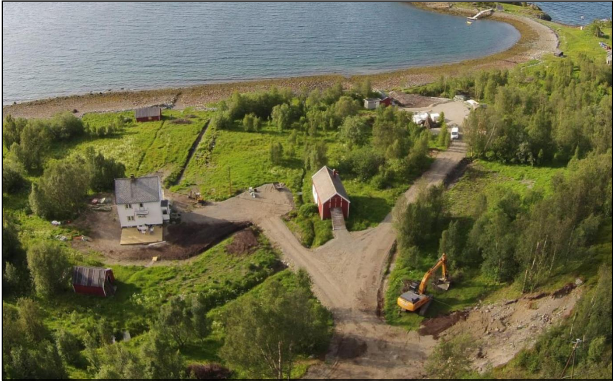
Figure 56: Bottom right corner shows where mass was removed. This mass was used for leveling the area east of the white house, and repairing the road. (Photo: Vidar Heitmann).
