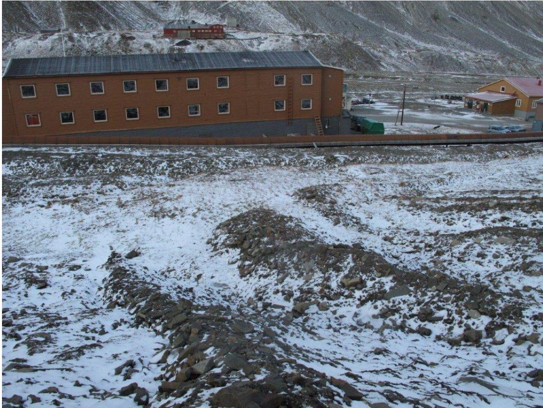
Figure 42: Debris flow Lyr14
