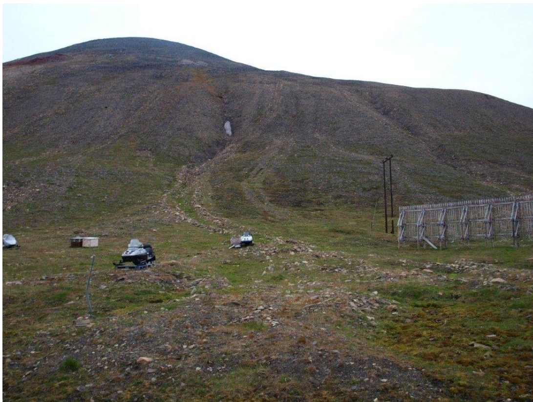
Figure 47: Runout of debris flow Lyr23
