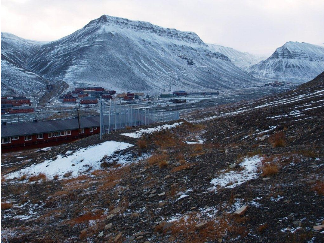
Figure 14: Trench, built in order to secure the kindergarten against snow avalanches and debris flows (Picture: Christian Engelke, September 2011)
